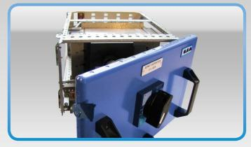
Possibility of performing infrared thermography measurements on functional units without power switch-off thanks to "open" position.
